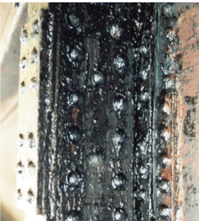
Removing resinated oil for renovation purposes
